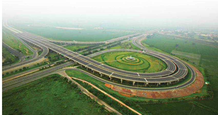
Fig. 4.7: Green Field Expressway
