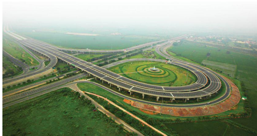
Fig. 4.7: Green Field Expressway
